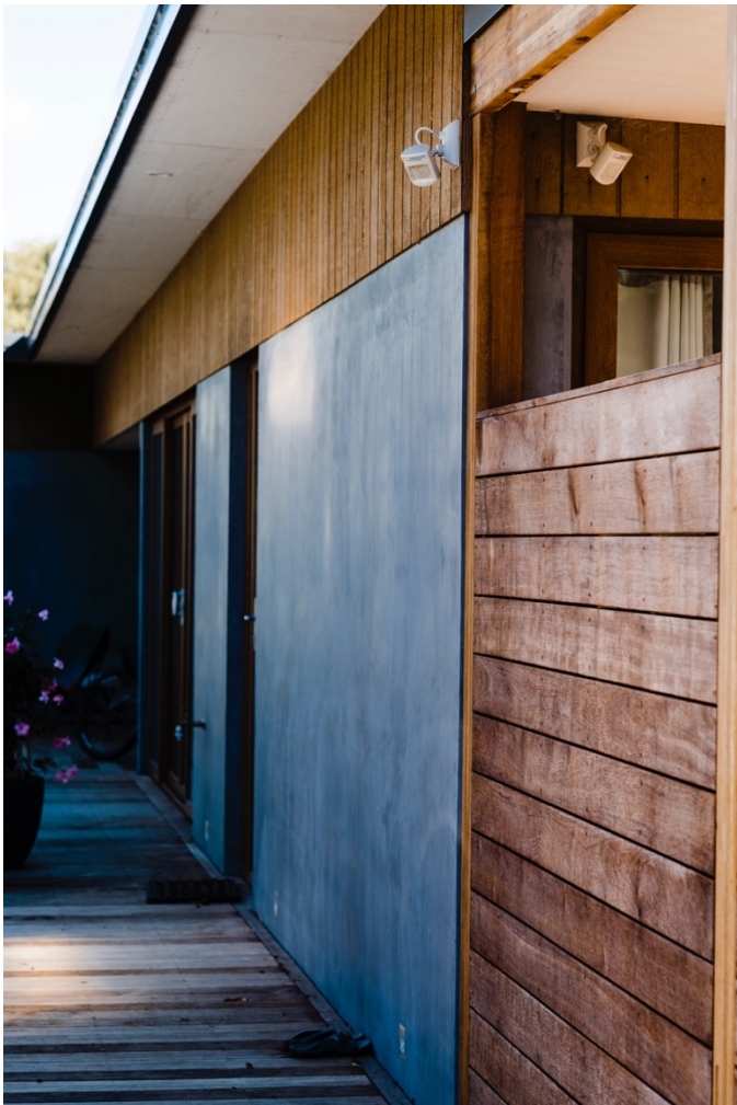
Figure 5. Witchcliffe hemp house, Hemp Homes Australia
