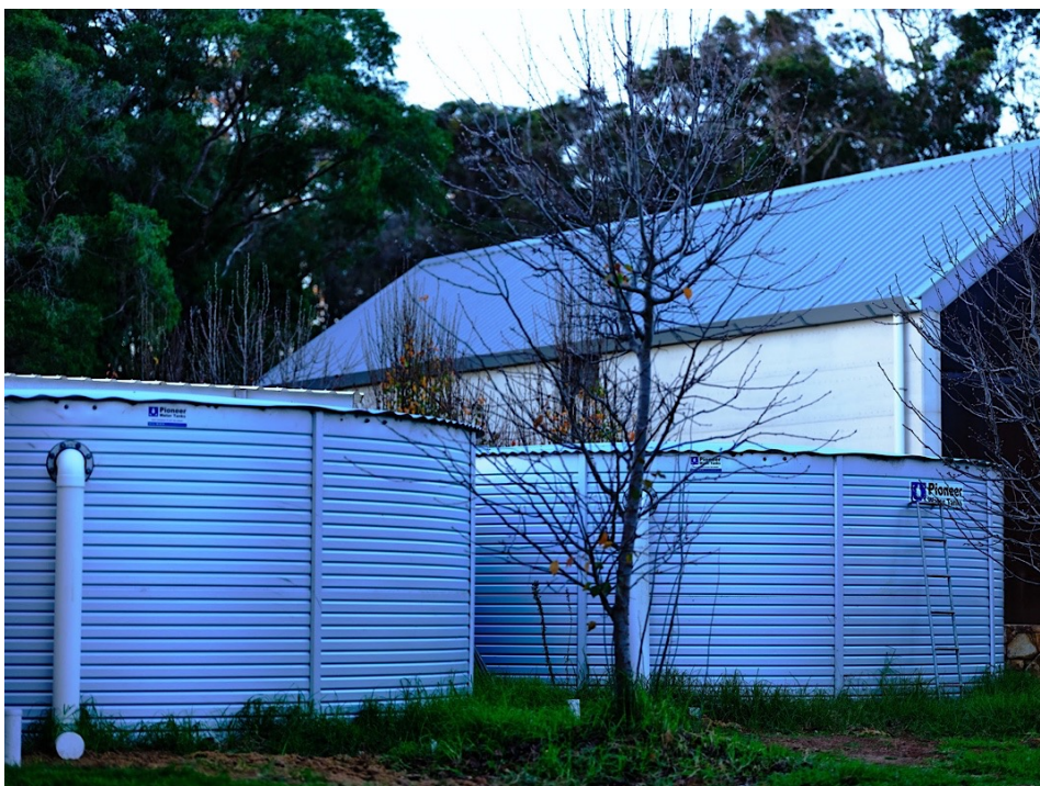
Figure 11. Rainwater tanks, Margaret River Econcepts house.
