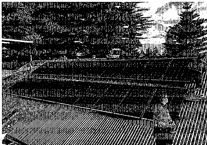
Figure 33. 6.4 kW PV array, Cottesloe
