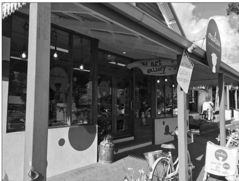
Example of a glazed shopfront building that creates a consistent street-edge, with a verandah extending over the public footpath creating enclosure and shelter
