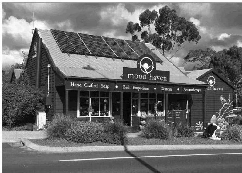
Well-proportioned, repetitive vertical windows sets up a pleasing rhythm along the street
