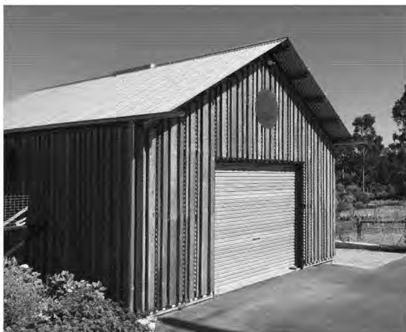
Figure 13. Modern rustic shed, Margaret River
