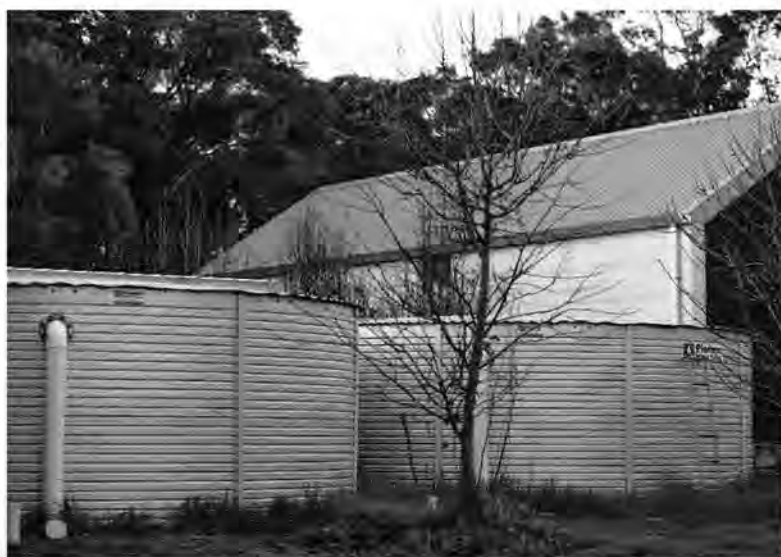
Figure 11. Rainwater tanks, Margaret River Econcepts house.
