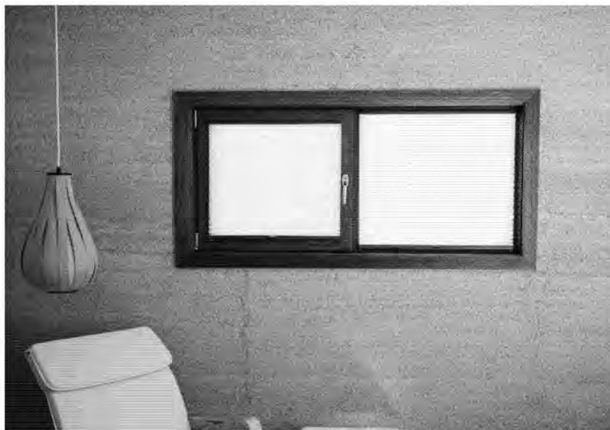
Figure 37. Margaret River hempcrete house, built by Hemp Homes Australia ( https://hemphomesaustralia.net.au/ )
